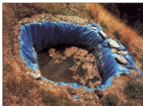
Fig. 8. Water stored in polythelene-lined tank
